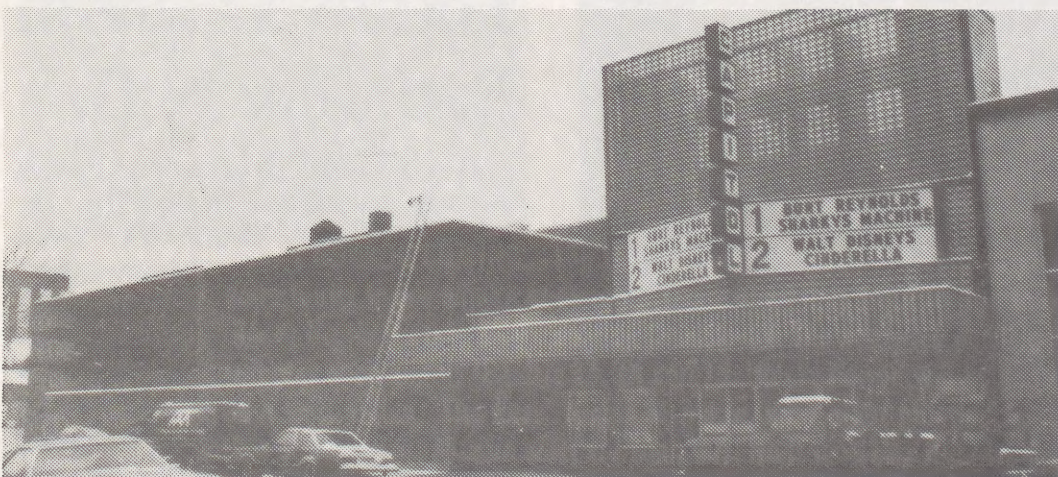
Outside view of the Capitol Cinemas showing newly constructed Cinema 2 on left with ladder.
